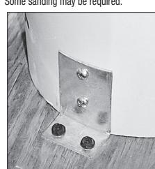
6. Mark and drill holes in floor and column shaft for corner/angle brackets (not included). (Column installation kit available #17040)
