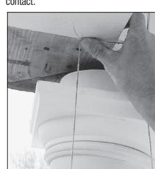
5. Put assembly in place and plumb. Make sure load is centered over column shaft and evenly distributed around the bearing surface.
