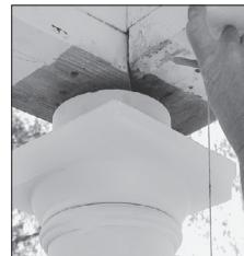
3. Slip base over top of column shaft and allow to slide to base of shaft. Slip cap over shaft and allow to rest on neck mould. Some sanding may be required.
