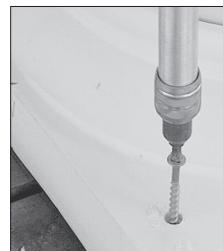
7. Apply construction adhesive\* to top of cap, press against structure, and screw or nail into place.
