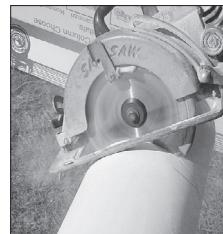
2. Use an abrasive saw (masonry or carbide tip blade). Fine trim top and bottom with rasp to ensure flat surface contact.
