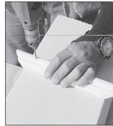
10. Pre-drill holes through neck mould into column. Screw neck mould in place or pre-drill and use finish nails.
