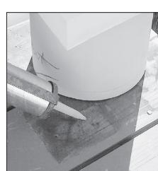
4. Apply construction adhesive\* to top and bottom surfaces of column.
