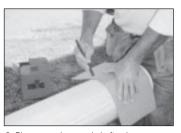
6. Place a mark around shaft using a straight edge.
