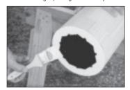
9. Paint the bottom end of shaft with a high quality exterior wood primer.
