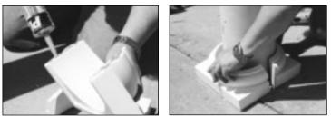
16. Apply construction adhesive to both cut edges of the split cap and split base. Nail or screw cap and base halves together. Caulk holes and where cap and base meet column shaft.
