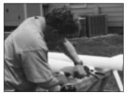
3.After cutting column halves to length, screw the aluminum flanges to the column approximately 2" up from where you cut the column off. Use your 1/8" diameter twist drill to drill holes. Use 3/8" diameter countersink bit to countersink the hole for screw. Install screw to secure flange.
