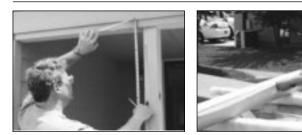
1.Measure the opening where column is to be used. Cut the column  $1/2^{"} - 1"$  shorter than the opening height. Measuring from the top of the column shaft towards the bottom, mark the column for cutting to length.
