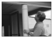
6.Set the column half with the aluminum flanges in place around the structural post. Slide the second column half into place, over the aluminum flanges, until the cut edges of the 2 column halves meet.
