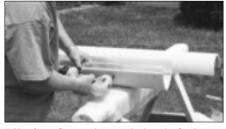
4.Aluminum flanges that run the length of column may have been fastened tightly to column for shipping. Use cordless drill and #2 Phillips driver bit, loosen screws fastening the 2 flanges to the column by approximately ¼". Pull each flange back away from inside face of column so there is a gap of approximately ¼" between the face of each aluminum flange and the inside face of the column.
