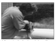
2.Separate the 2 column halves. If purchased pre-installed, aluminum flanges will be attached to one of the halves. Place edges down. Cut each shaft half to length with carbide tipped blade. Carbide blade will cut fiberglass and aluminum. Slowly cut through the (2) aluminum flanges as you cut the column shaft to length. (see Note 1)
